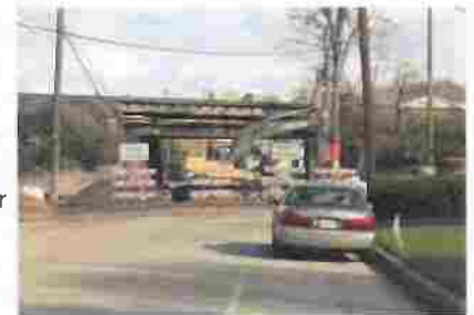
Sinkhole Remediation Project on Butler Pike
